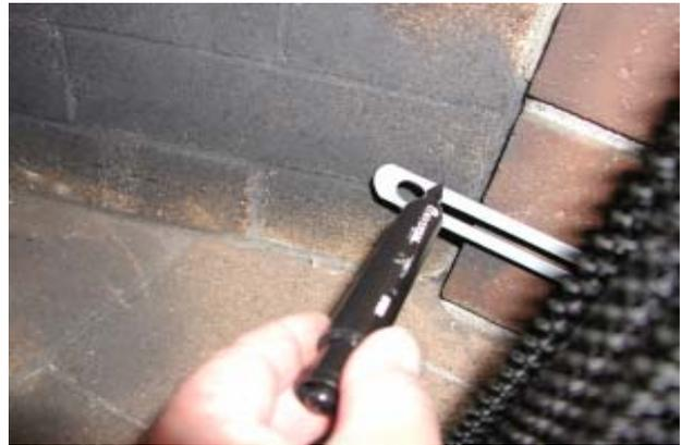
**STEP 6** Using a 5/16" masonry bit, drill hole where marked.
