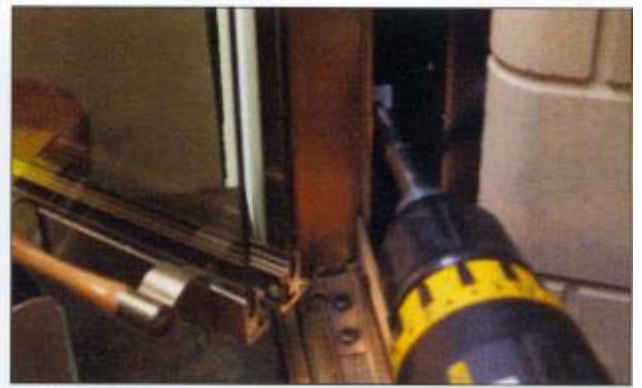
STEP 11 Gently open left door ( Do not move alignment ), and install self drilling screw . Close and recheck alignment. Repeat Step 11 on right side.
