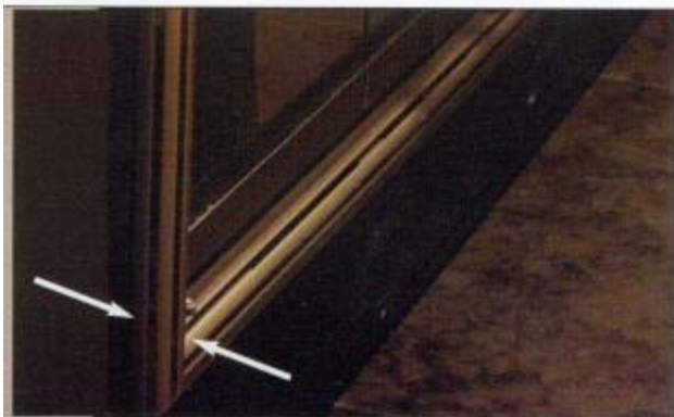
STEP 10 Move bottom of door in or out to align top face of doors.
