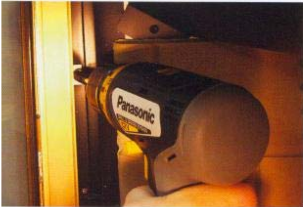
STEP 8 Screw into position at top left. (Note: Make sure frame does not move. Screw into position at top right. Do not over tighten, this may strip out screw.
