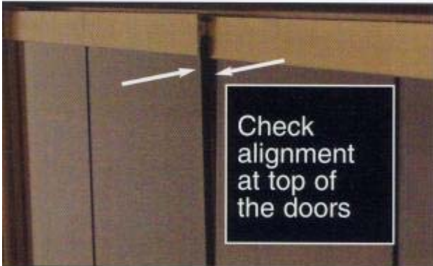
STEP 9 Check alignment at top of doors. Note: magnets hold doors at bottom in alignment. If alignment is needed at top of doors see Step 10.
